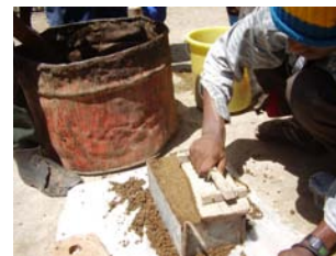
Step 2. Compacting
