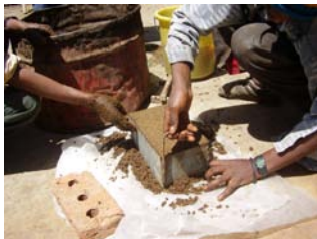
Step 3. Opening the mold
